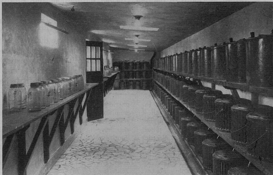
Figure 2. Inside view of lysimeter
